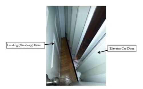
The above picture shows a Residential Elevator with Space Between the Exterior Swing Landing (Hoistway) Door and Interior Elevator Car (Accordion) Door. A young child can become entrapped if there is an excessive space between the doors.
