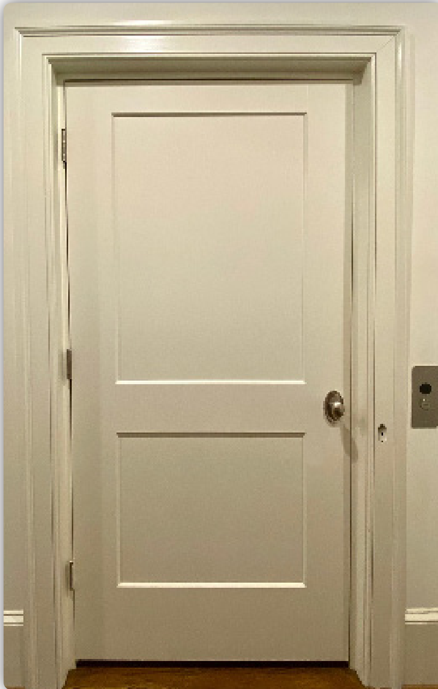
Flush door frame with key cover (door and frame by others)
