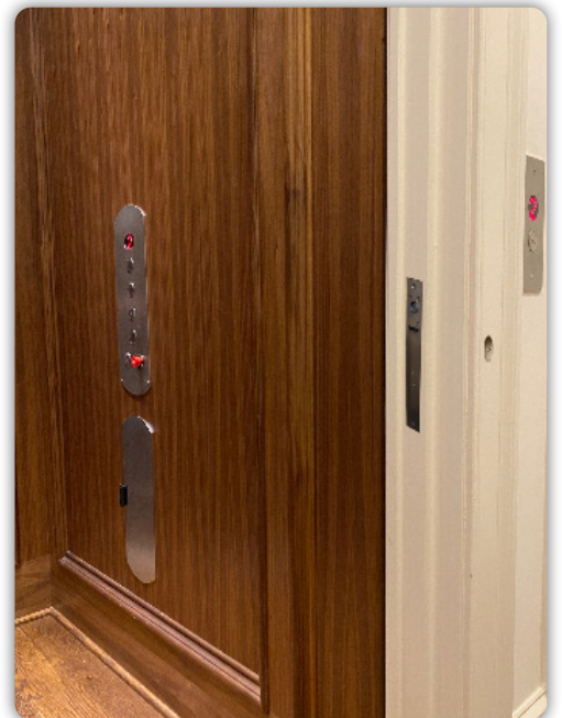
Symmetry Locking Device mounted in door frame
